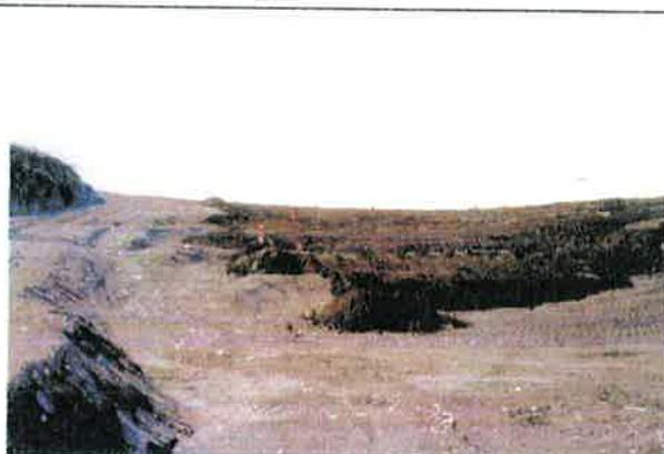
**Photo 8-13 Topsoil placed on clay barrier to prevent desiccation cracking, Penticton B.C Fire.**
