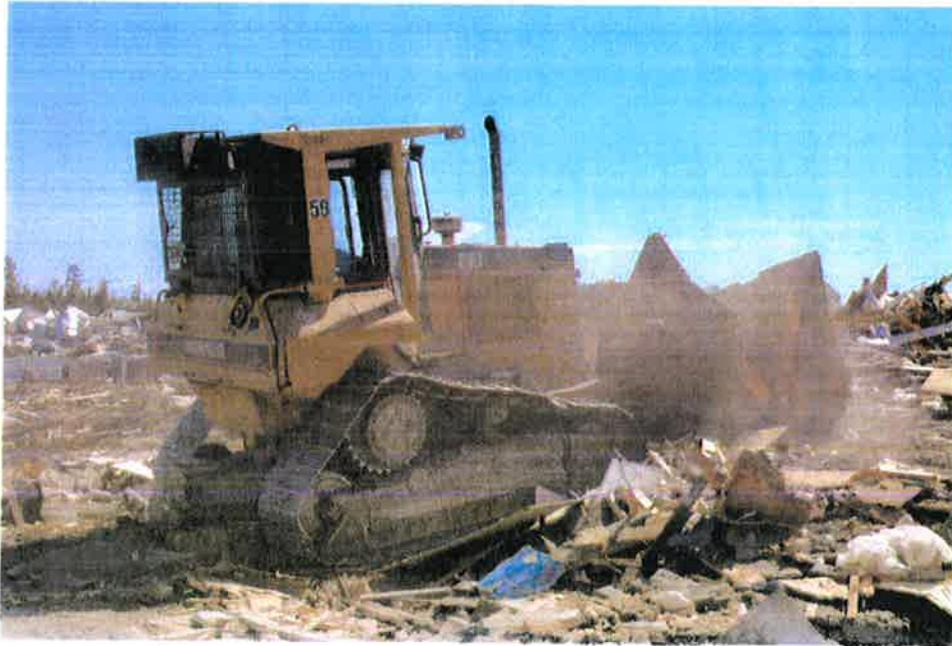
**Photo 11-2 Bulldozer Compacting C&D Waste**
