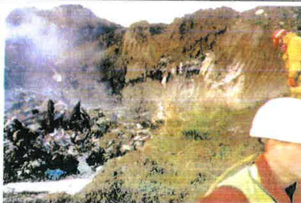
Photo 8-3 Spontaneous Combustion, Closed Landfill in Delta
