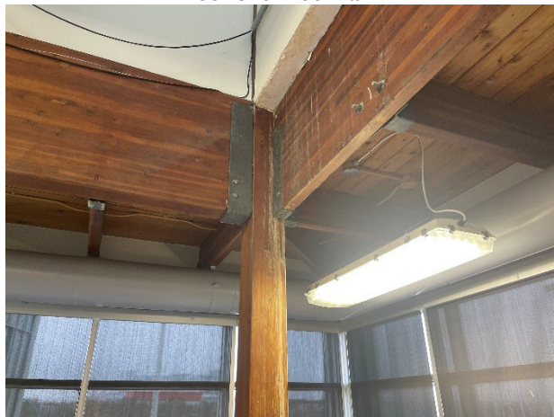
Roof Over Pool Tank
