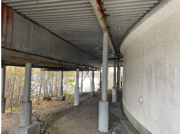
Rear Deck Foundation Piers and Columns
