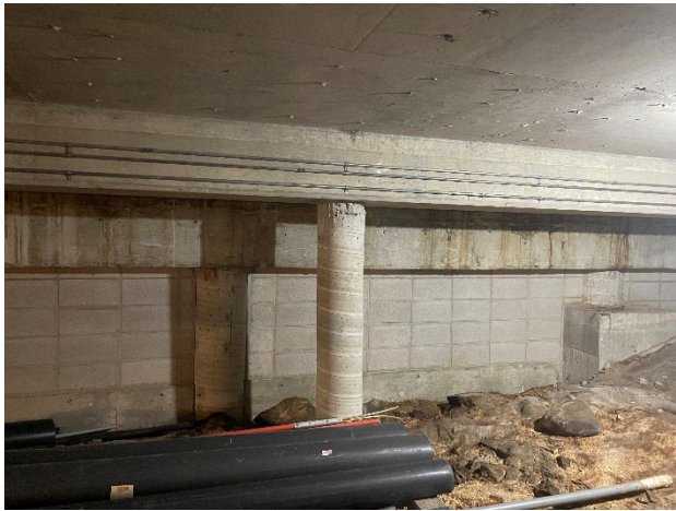
Underside of Main Floor in Crawlspace
