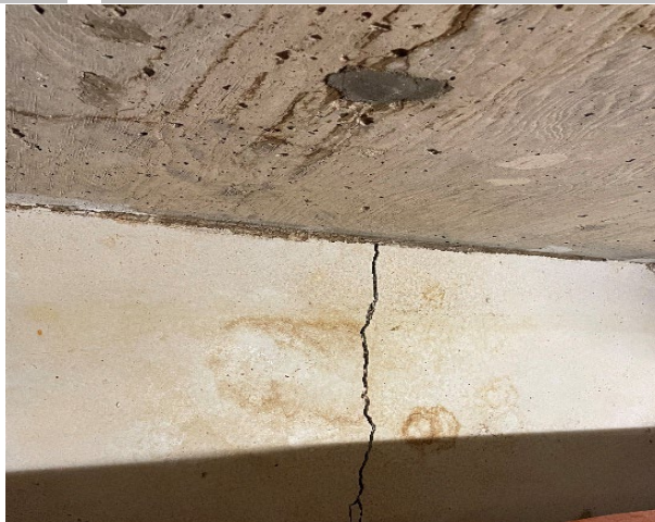
Basement Floor Slab Around Base of Pool Tanks
