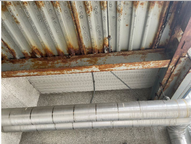
Underside of Rear Exterior Deck
