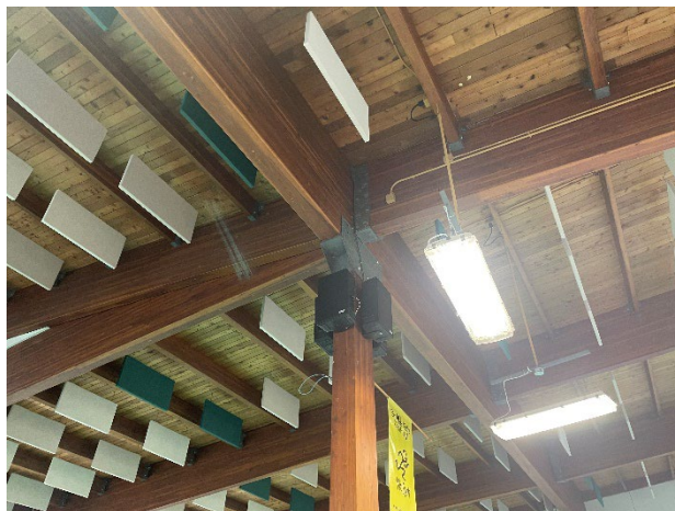
Roof Over Pool Tank
