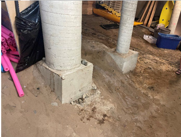
Crawlspace Foundation Piers
