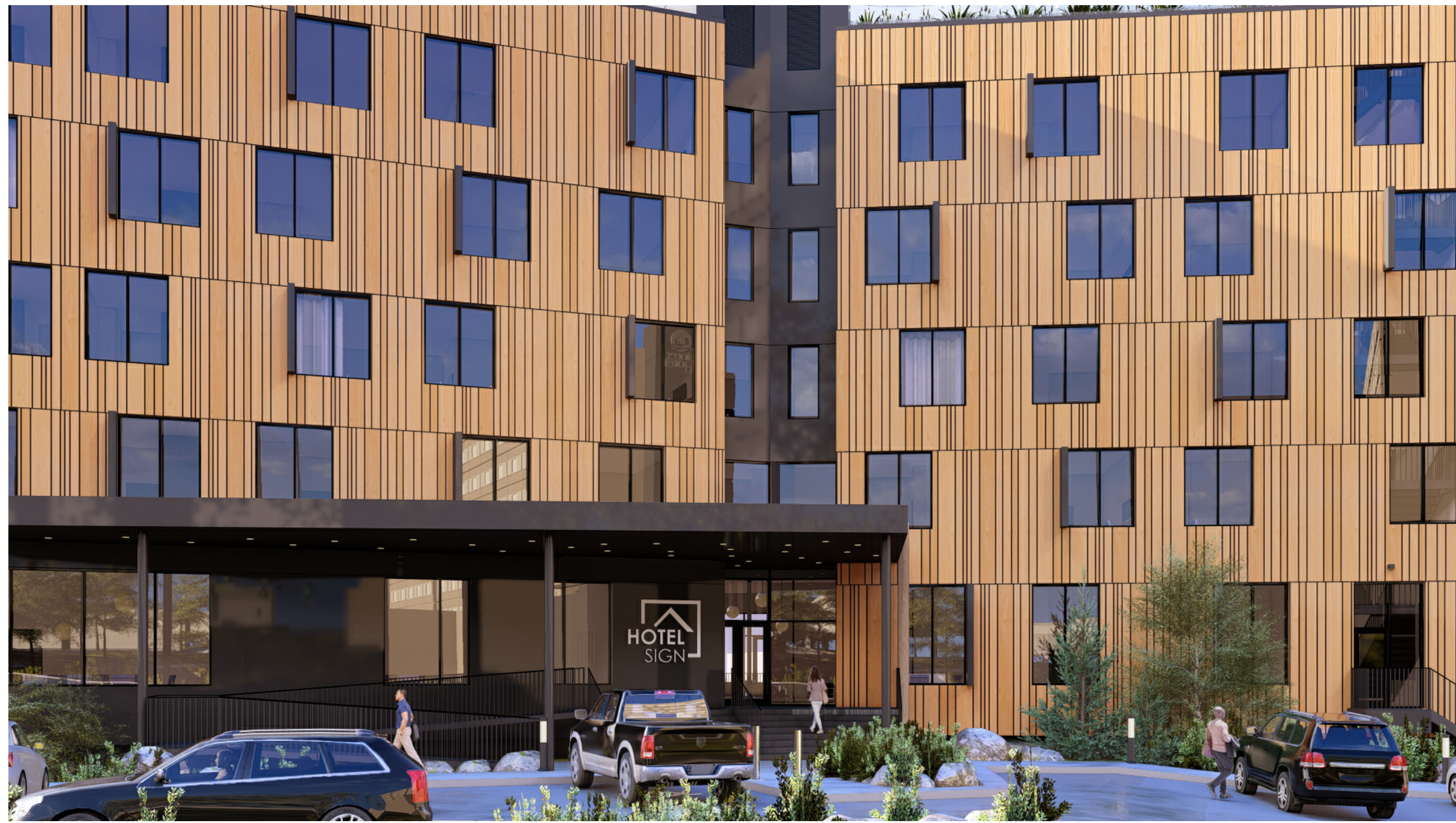
VIEW OF THE HOTEL ENTRANCE
