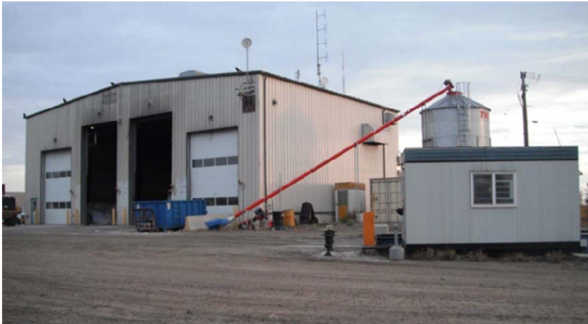
Photo: Photo of the Bailing Facility and Gatehouse at the Solid Waste Facility.
