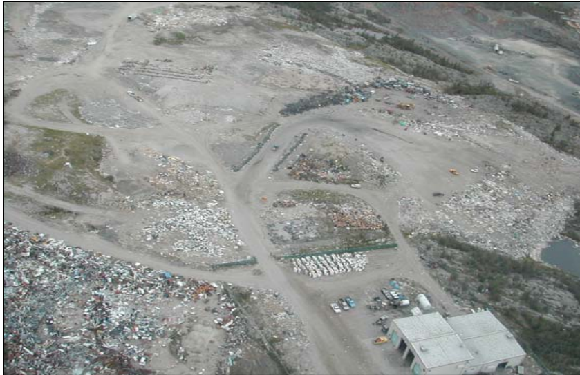
Aerial View of the Solid Waste Facility
